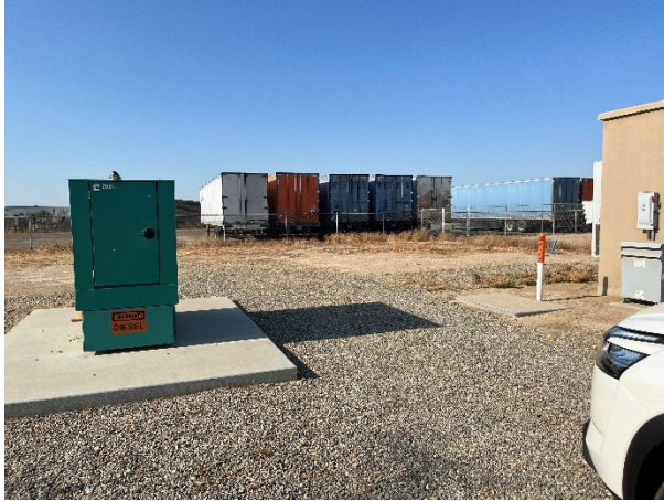
Figure 3. Headend Backup Generator
