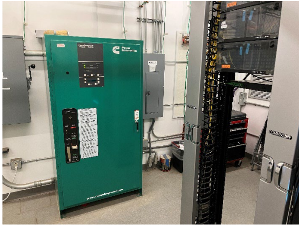
Figure 7. Automatic Transfer Switch
