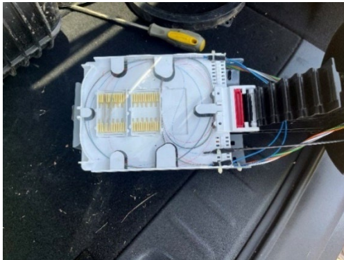
Figure 22. Splicing Tray 2
